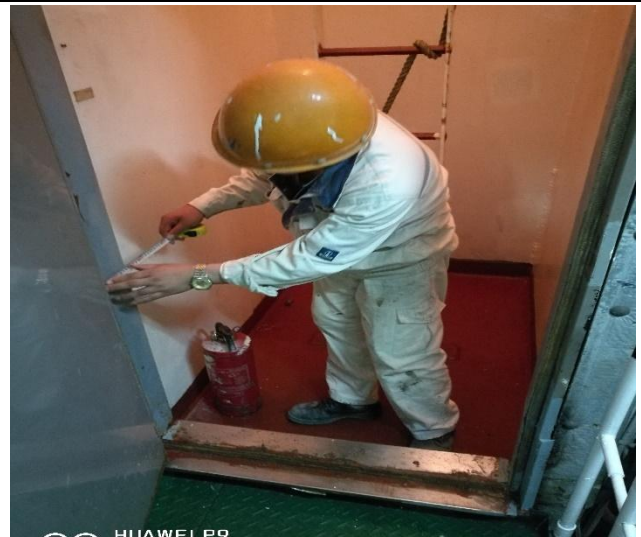
Measuring fire door for new fabrication
