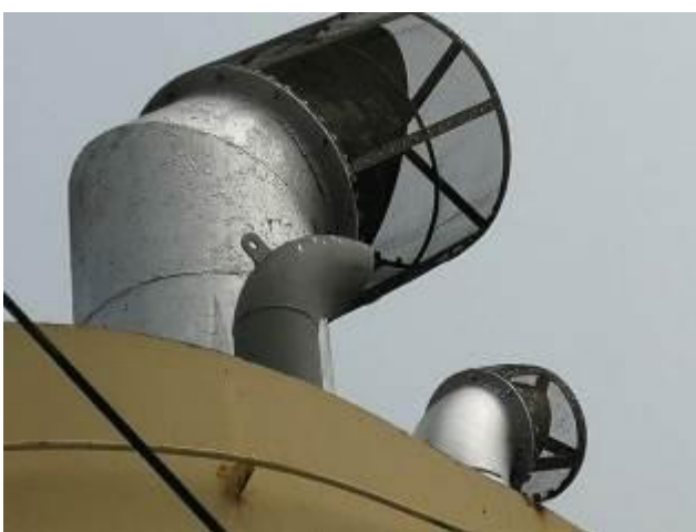
Spark arrestor fabricated and installed
