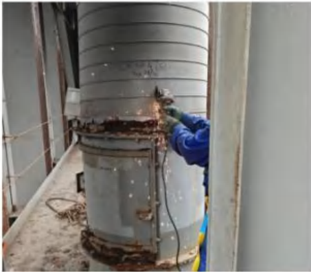
Cargo hold ventilation ducts replacement service
