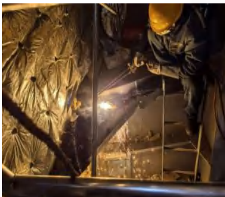
Main Main engine insulation rectification service
