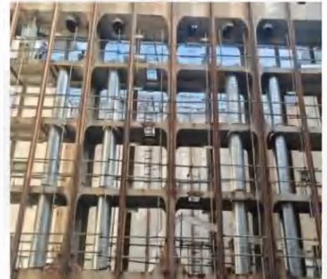
Cargo hold ventilation ducts replacement service
