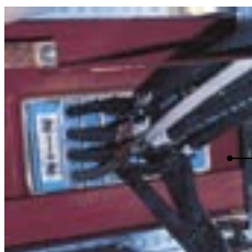
Roxtec installation in switchboard.
