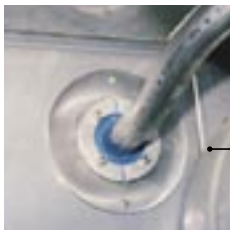
Roxtec RS seal for sprinkler system in kitchen.
