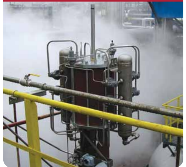
SVI II AP on steam conditioning valve
