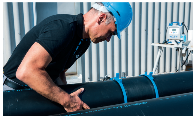
Slide both ends of the pipe into the fitting as far as the marking. Then remove the assembly aid.
