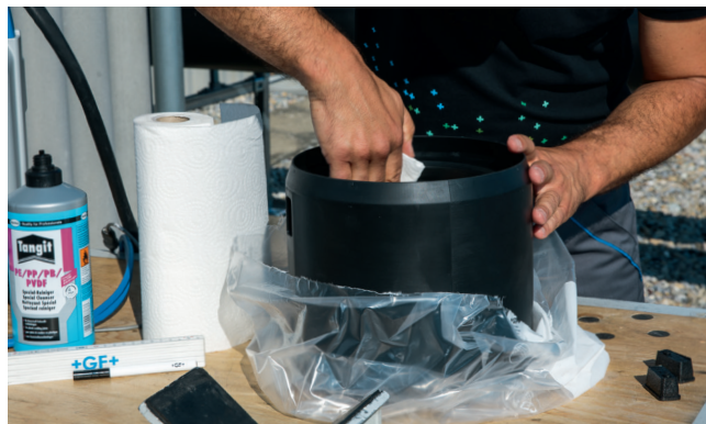
Clean the fusion zones of the fitting and pipe using Tangit PE-cleaner and a clean paper towel.
