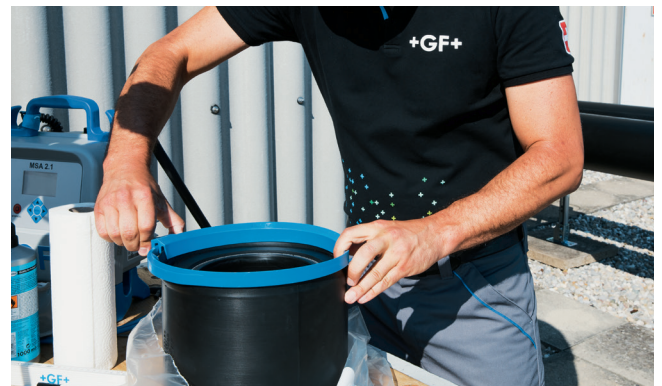
Place the assembly aid on the fitting. Stretch the sealing lip pressing the handles together.
