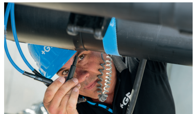
Connect the welding cables to the welding contacts of the fitting and weld according to the instruction manual.
