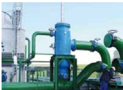
24" / DN 600 FTAF Filter Bioethanol plant
