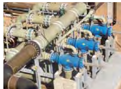
3 x 16" / DN 400 FTAF Filter desalinisation
