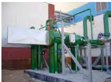
24" / DN 600 FTAF Filter seawater cooling
