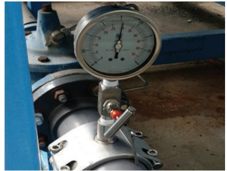
MJD-A EPDM 100mm. pressure gauge installed on PVC pipe. water supply line at power plant. Thailand
