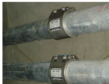
MJGF EPDM 100A. drain pipe. subway station. Japan
