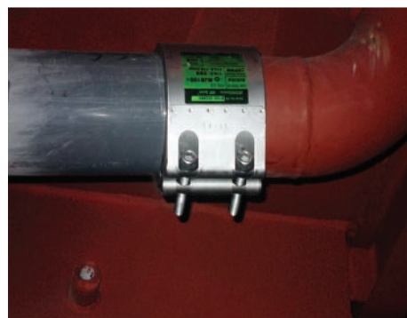
MJS EPDM 100A. PVC pipe + steel pipe. Korea
