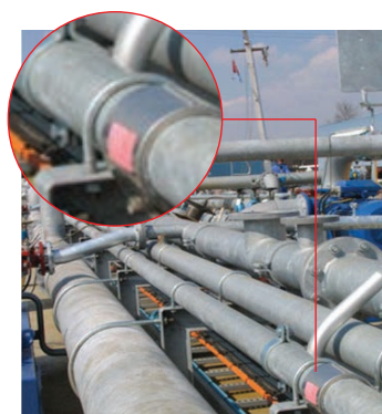
MJG EPDM 100A. sprinkler line for deck wash. Netherlands
