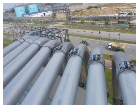
MJG. silo system.
