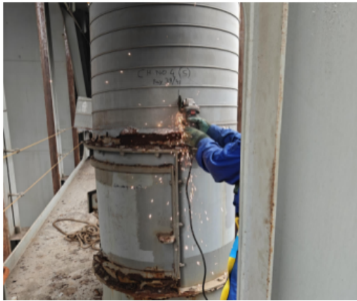
Cargo hold ventilation ducts replacementservice
