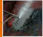
Surface - Sand blasting
